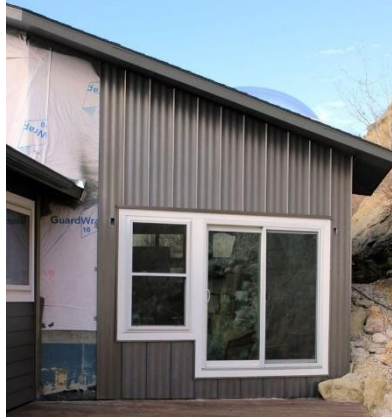
Steel Siding, Non-corrugated Figure
